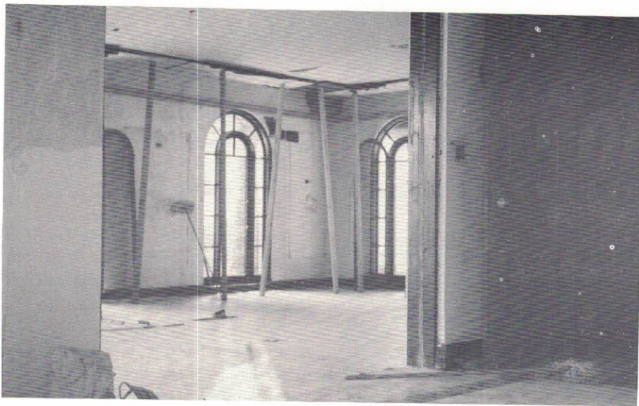
Terrace Villa "insides" thrown out! New interior takes shape.
